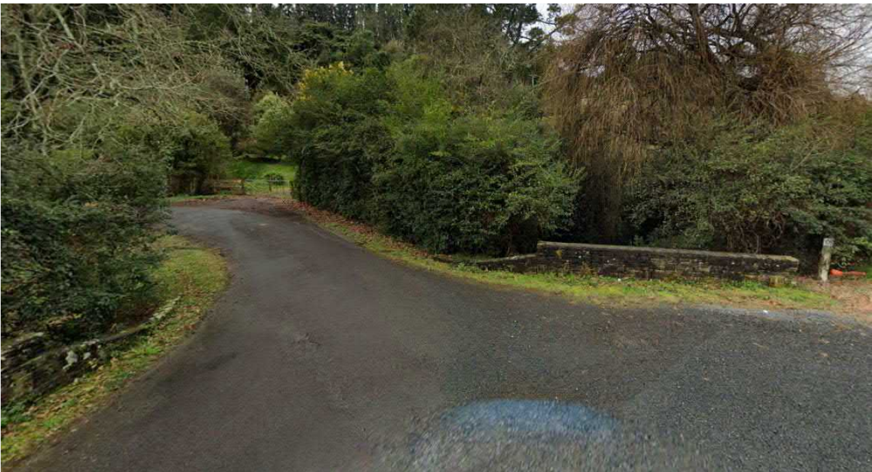
Figure 16: Formed Access to Existing Properties within the Site
