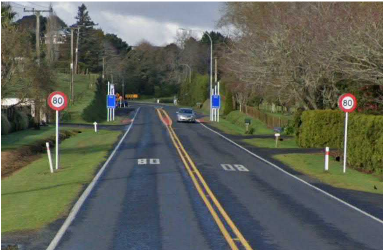
Figure 13: Facing south on Oropi Road
